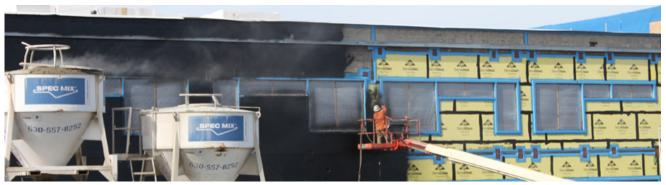
Workers apply a vapor barrier to the east side of the Phase I building at the Riverfront Campus. This coating will help to seal the exterior.
