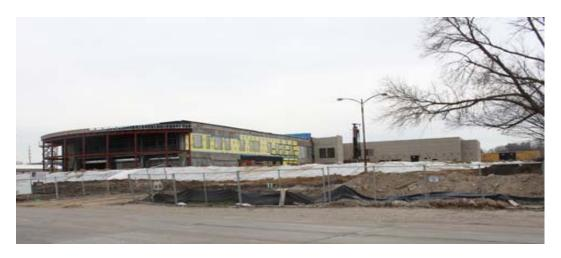
(A view of the northeast corner of the building, which shows the berm built for flood protection.)
