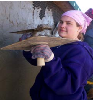
Autumn Campbell doing stucco
