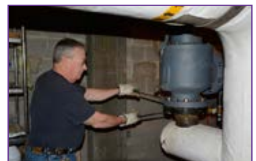
Repairs being made during the annual steam system shutdown.
