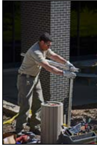
New cable guard rail at the south entrance to the Union.
