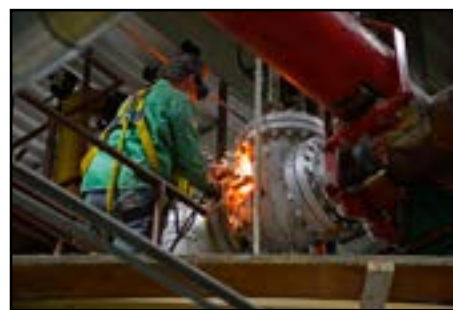
Repairs being made during the annual steam system shutdown.
