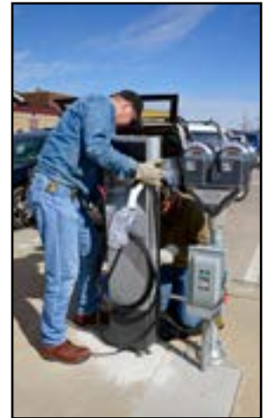
New electric charging station being installed in Q-lot.
