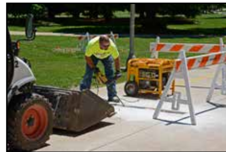
Repairing sidewalks around campus.
