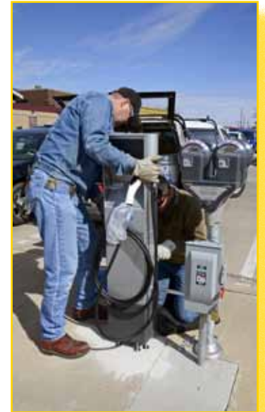
Charging Station Installation
